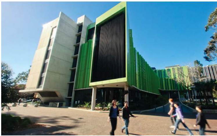
Entry vial UNSW Gate 10
